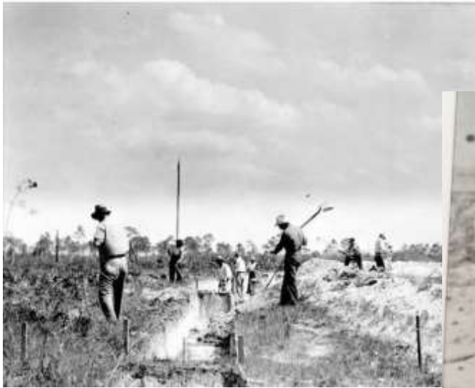
Construction by the FERA of north River Road between Alva and Olga - Lee County, Florida 1935
